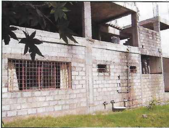
Kashmir Bhavan under construction
