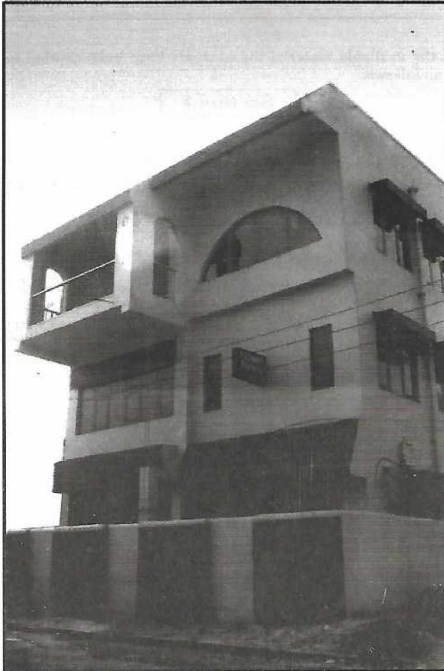
Kashmir Bhavan Building Kashmir Sabha, Kolkata CK-35, Salt Lake City, Karunamoyee, Kolkata-700 091
