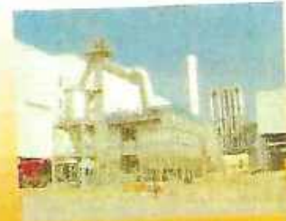
De-Dusting System for Steel Melting Shop, OMAN
