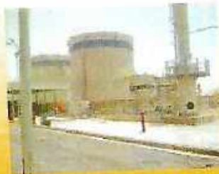
Fuel Oil Handling - Saudi Arabia
